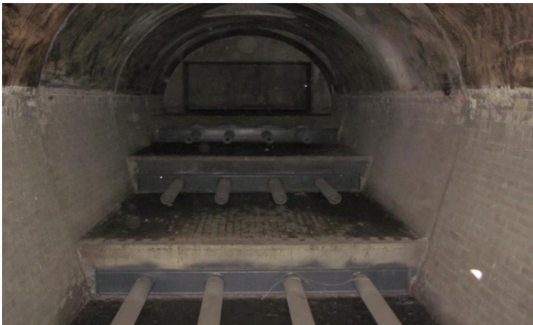
Inside the 100 Ton Incinerator.
